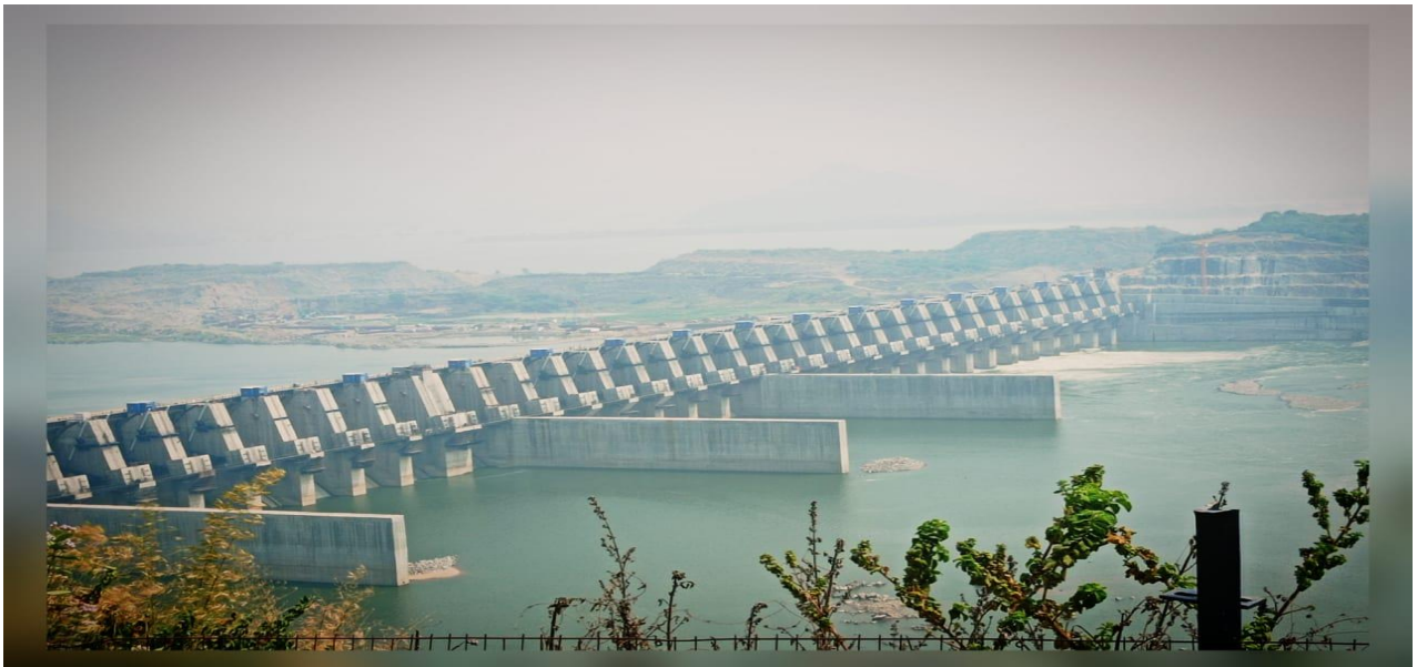
CONSTRUCTION SITE VIEW OF POLAVARAM PROJECT
